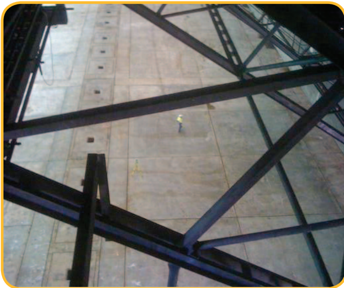
Part of sugar shed roof structure
