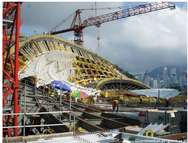
The iconic roof of the West Kowloon Terminus and its complex steel structure. Image captured onsite, during the installation and erection of the steel structure in June 2017.
